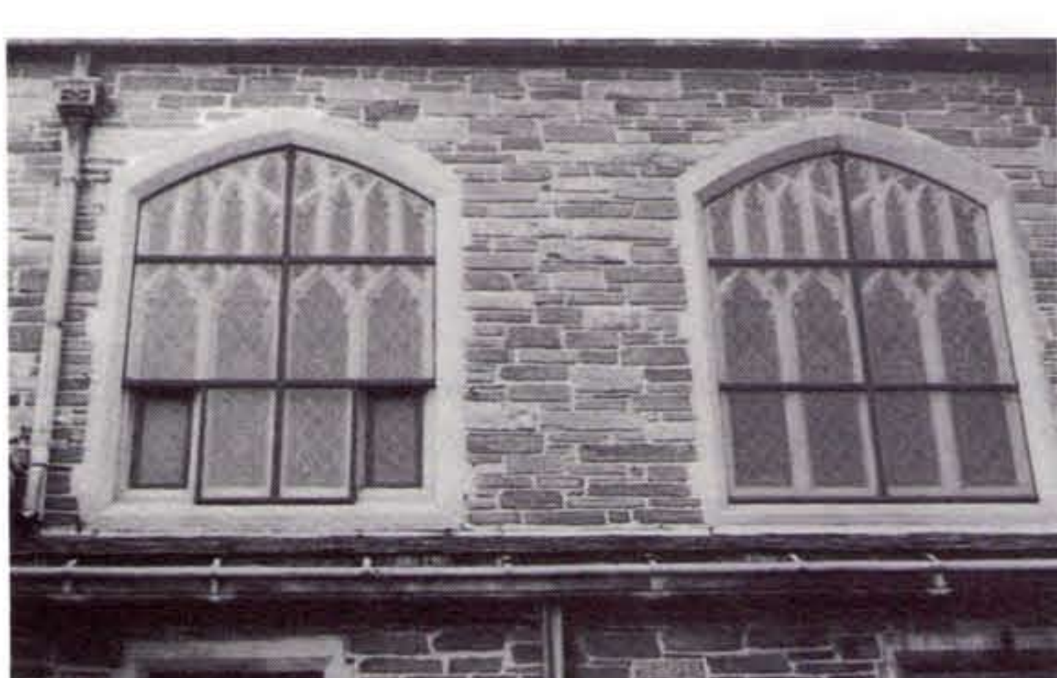
Cathedral Stoneworks is replicating a total of 34 Gothic-style limestone tracery windows.
