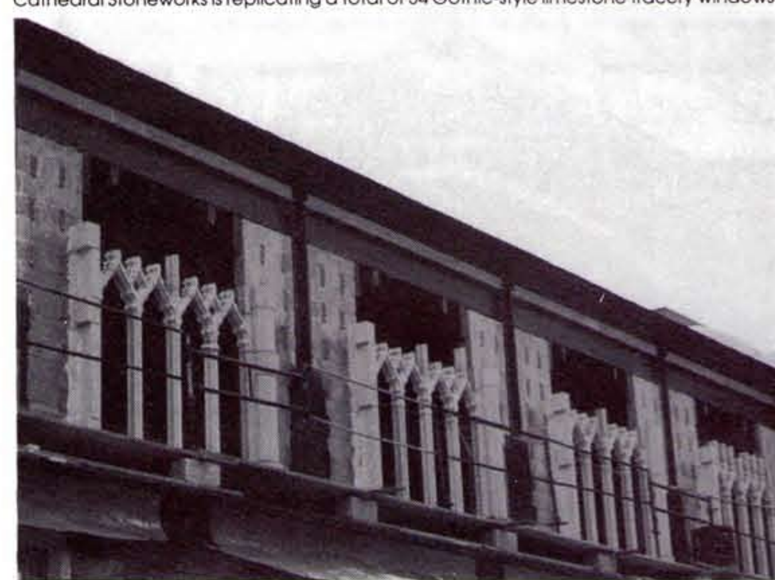
Cathedral Stoneworks is replicating a total of 34 Gothic-style limestone tracery windows.
