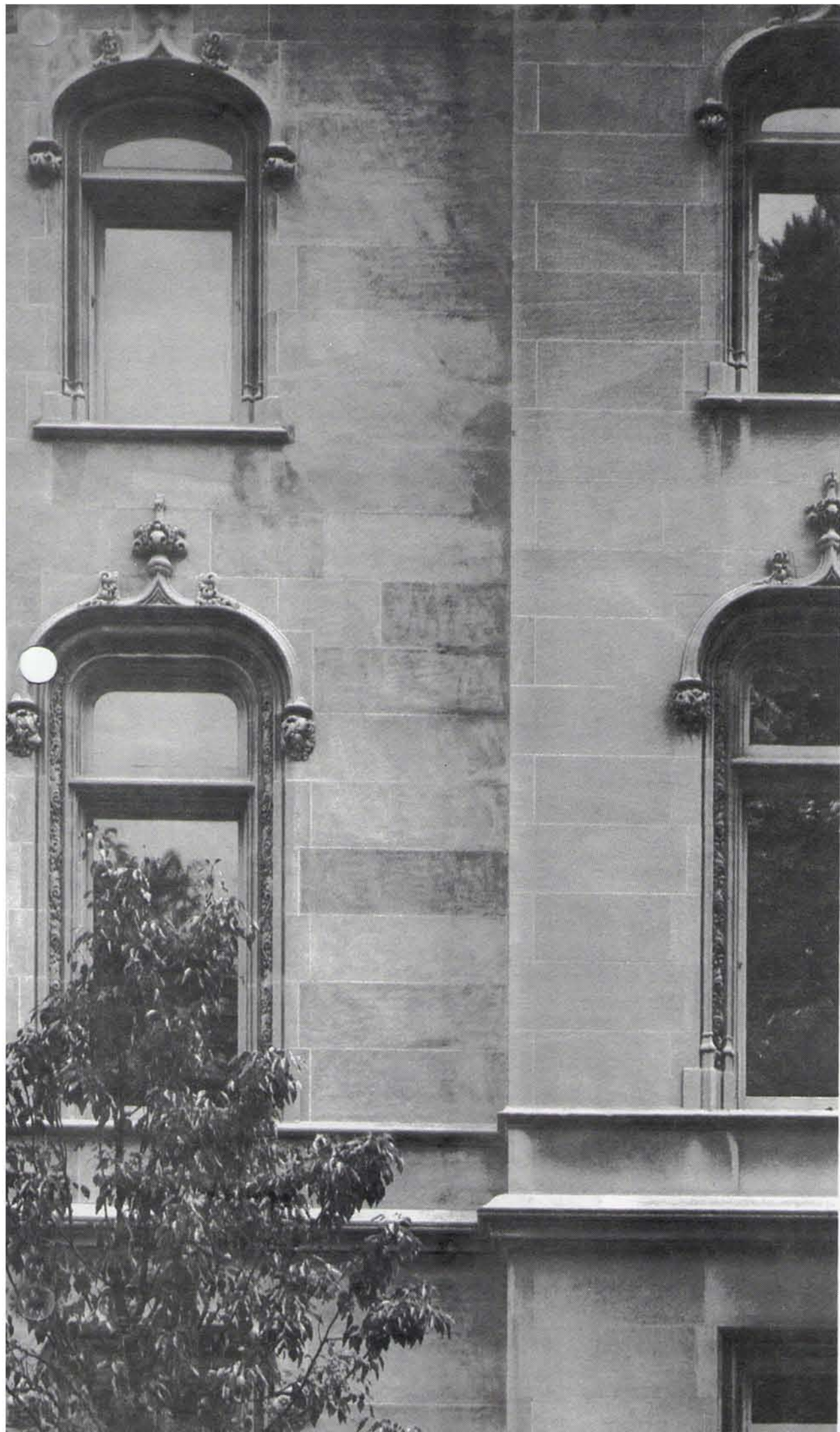
FACING PAGE: The carved stone facade of the Roche addition is supported by a steel frame with concrete floor plates. LEFT: The bay of the new addition (left) is almost indistinguishable from the 85-year-old original (right). TOP: Workers hand-chiseled the surface of the new limestone to simulate the effects of weathering on the original. CENTER: As required by the New York City Landmarks Preservation Commission, a balcony removed from the Warburg Mansion's rear facade was reinstalled on the Fifth Avenue elevation of Roche Dinkeloo's addition. ABOVE: The preservation commission also required that new window moldings exactly match the originals.
