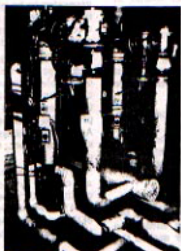
FUEL AND SPACE SAVER , the Hitachi chiller/heater (top) installed at 111 Fourth Ave. saved $56,211 in fuel costs in six months. The unit occupies 2,503 cu. ft. The former HVAC system boiler (above right), hot water (above), chiller (right) and condenser (not pictured) took up a total of 12,610 cu. ft.
